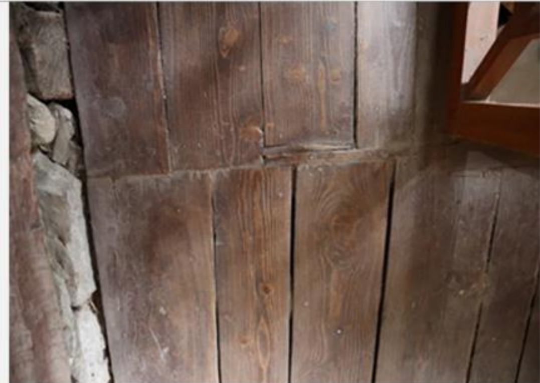
Floor are made of wooden batterns of approx. 100mm x 700mm
