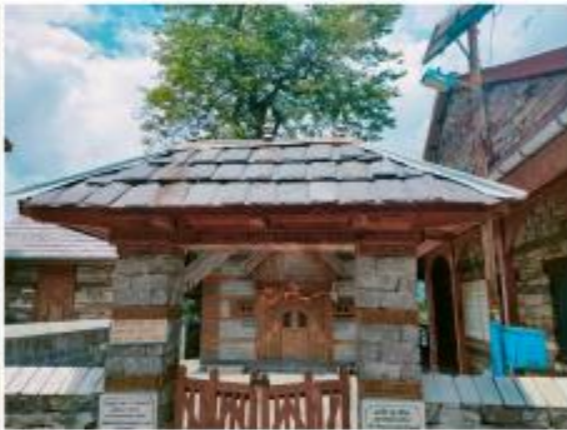
Slate tiles used to protect the structure from rainfall and snow
