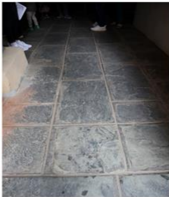
The basement floors are of stone tiles of 600 x 600mm
