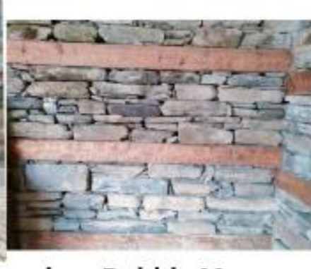
Random Rubble Masonry
