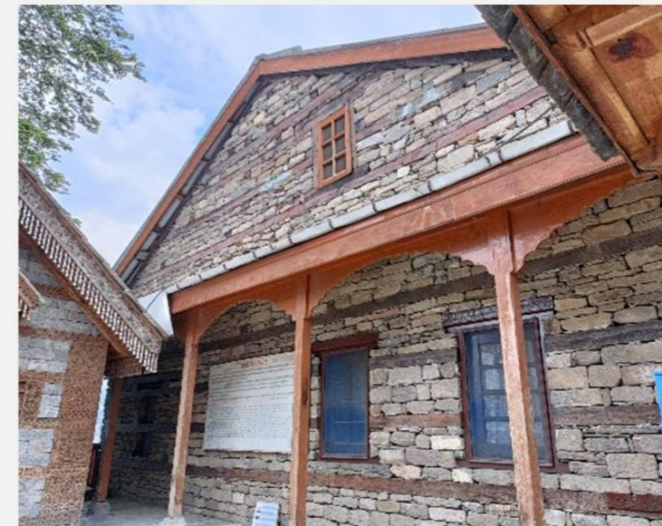
Gable windows are provided for light and ventilation.
