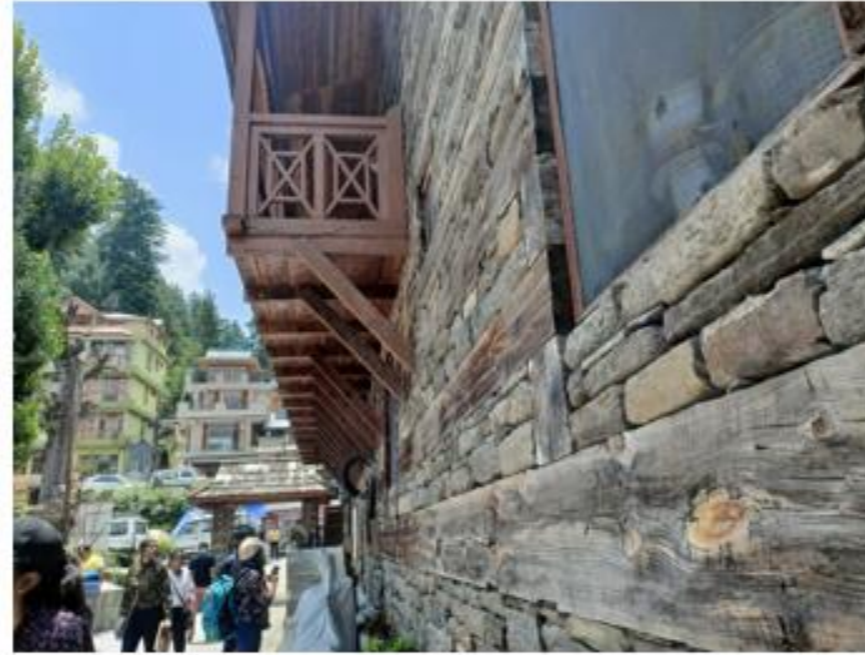
Wooden trusses supporting the balcony.
