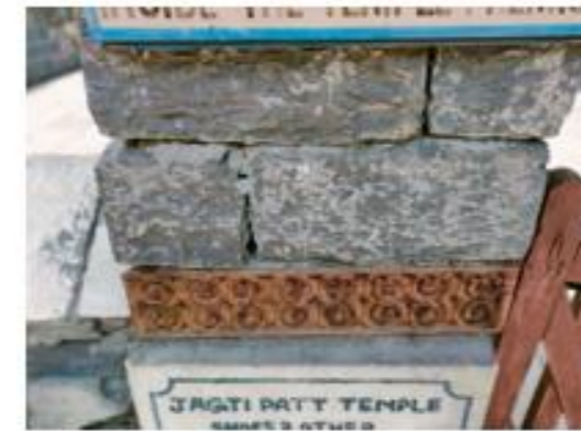
Random Rubble Masonry
