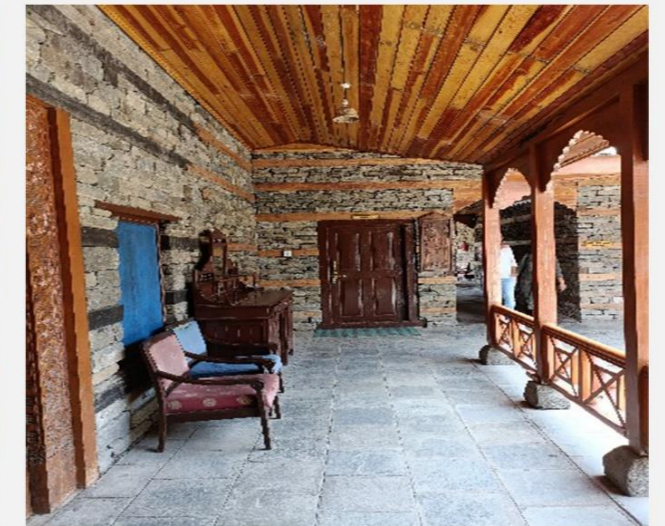
On the ceiling wooden planks are used as false ceiling.
