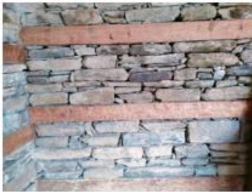
Random Rubble Masonry
