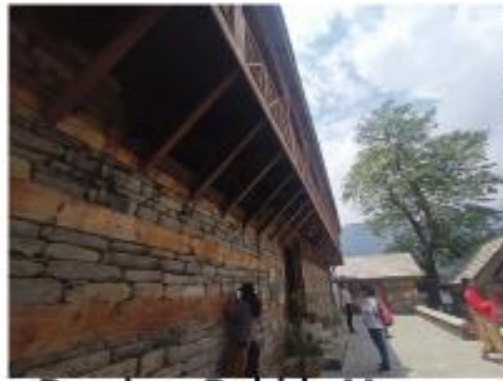
Random Rubble Masonry
