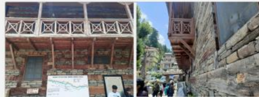
Wooden trusses supporting the balcony.
