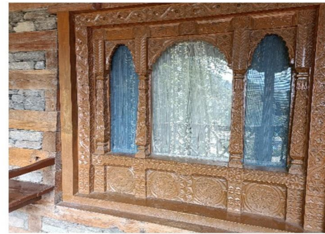
windows with low sill height and heavily carved.
